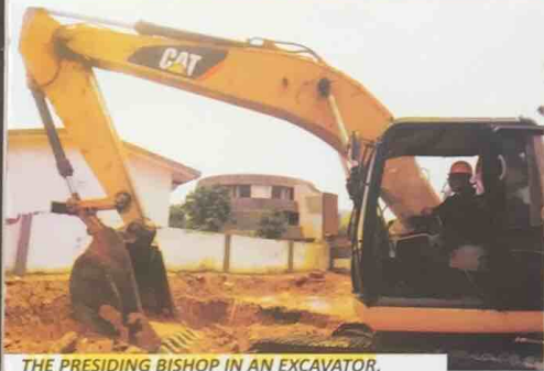
THE PRESIDING BISHOP IN AN EXCAVATOR, BREAKING GROUNDS FOR WORK TO COMMENCE
