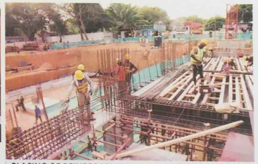
PLACING OF REINFORCEMENT IN THE GROUND FLOOR SLAB
